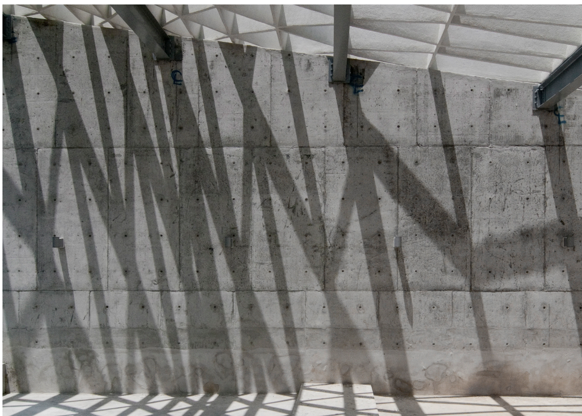
06: Façade Pattern on North East Elevation; A Simple Factory Building , Singapore, 2008-12.
