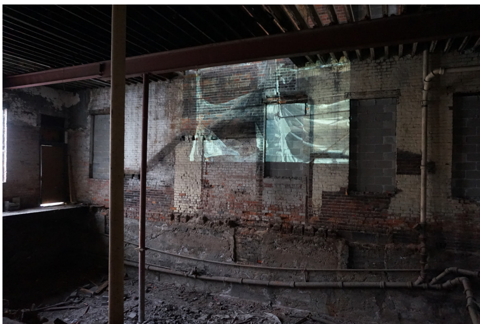
02: Plastic and scaffold in derelict carriage factory, Iowa's Ohio.
