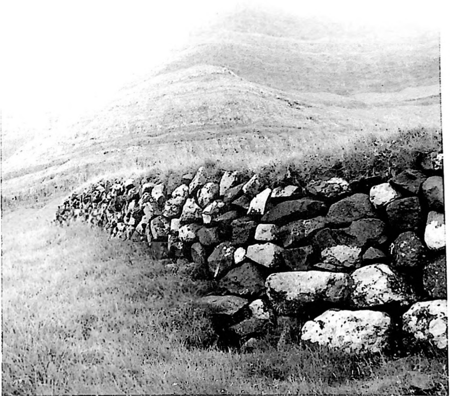
Fig. 4 The wall which, during the round-up, guides the sheep into the fold in Múli's infield. The wall is built with a 'chest' and 'back': a steep, stone side out towards the sheep and a sloping, grassy bank on the other side. Photo 1961.
