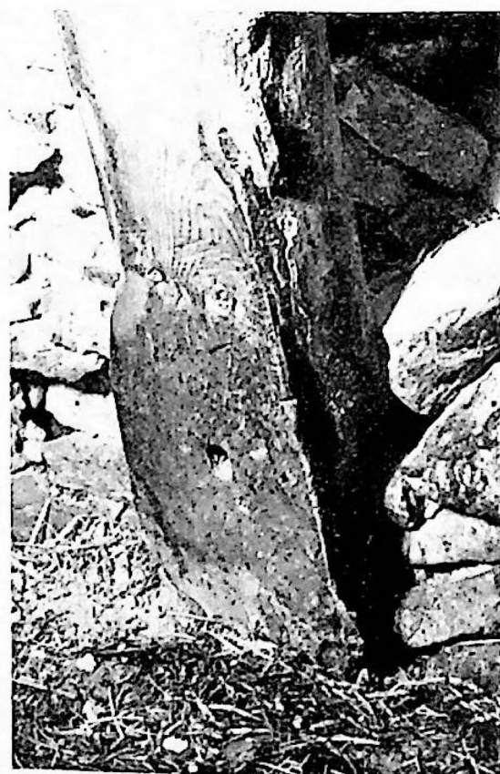
(above) cruck base and mortice-hole (NW blade, cruck v) (left) collar-joint and bracing peg (NW blade, cruck III)
