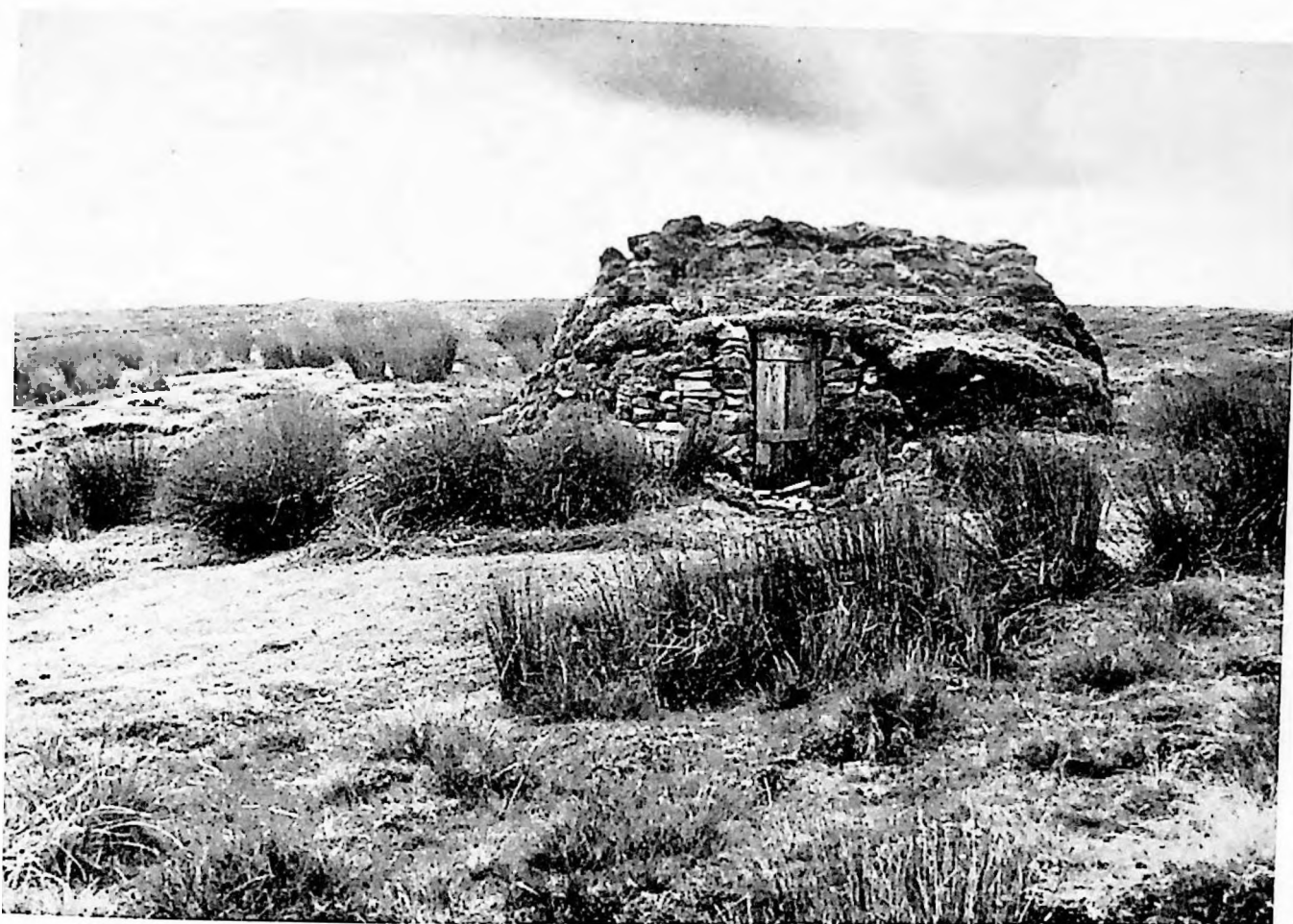
PLATE V. Traditional type of shieling hut NB 388436, 500 yards west of A857, 7 miles from Stornoway. This and two similar but roofless bothies stand on grassy slopes of a burn incised into calluna moorland on deep peat. Inside dimensions 6 ft. by 10½ ft. walls c. 5 ft. thick and 5 ft. high inside, slightly higher and stone-built on outside at the door. Otherwise the outside walls banked up by peaty turf. Roof of drift wood covered with tarred felt and some corrugated iron sheets and overlaid by thin inverted grassy turfs. A square foot of glass in roof for skylight. To the right of door on entering, a wooden bench c. 6 ft. long and on opposite wall a wire spring bed c. 6 ft. by 3½ ft. supported on stones and with a mattress of heather bushes. Very well-built interior walls with two inset 'cupboards' 1½ ft. by 1½ ft. and several layers of wallpaper on walls. Open fireplace in end wall on left of door with old bottomless enamelled cooking pot (visible on left peak of roof ridge) as chimney. Wooden cupboard with cups, oil lamp, etc. on back wall by fireplace; a brander for oatcakes. (Photographed in August 1966). (See page 193.)
