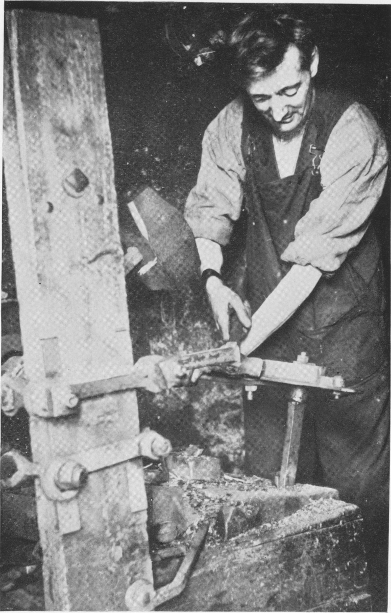
Making a "hold-fast" at the "oliver". (See p. 118).
