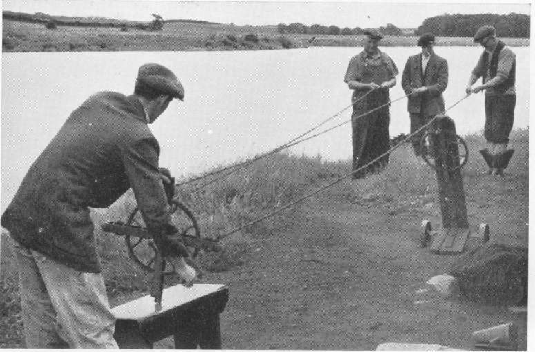
FIG. 1—Twisting the strands (see p. 117).
