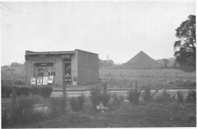
FIG. 2.—Recent building. A shop at west end of village, Ormiston.
