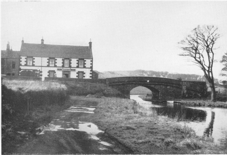
FIG. 2.—Canal and bridge, Ratho.
