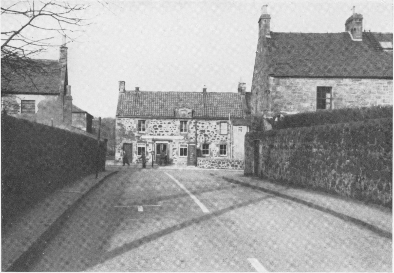
FIG. 1.—Entry from south, Ratho.
