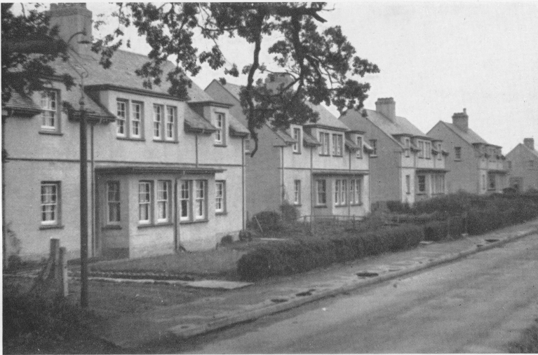
FIG. 2.—County Council housing, Ormiston.
