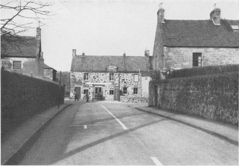
FIG. 1.—Entry from south, Ratho.
