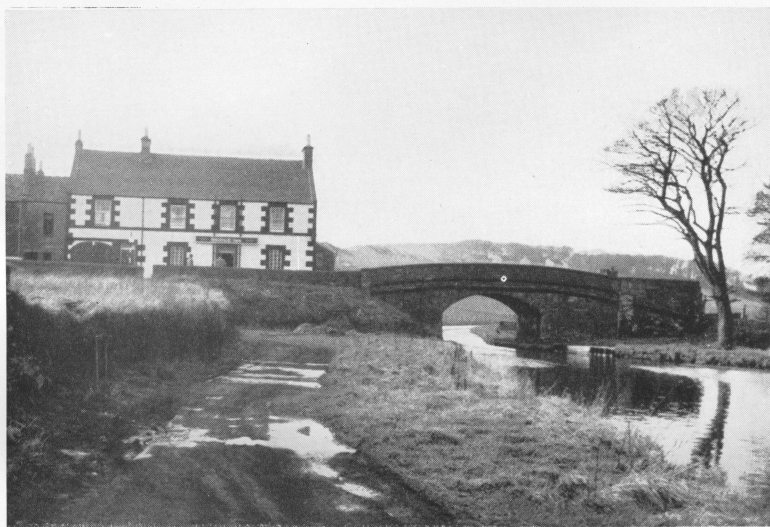
FIG. 2.—Canal and bridge, Ratho.
